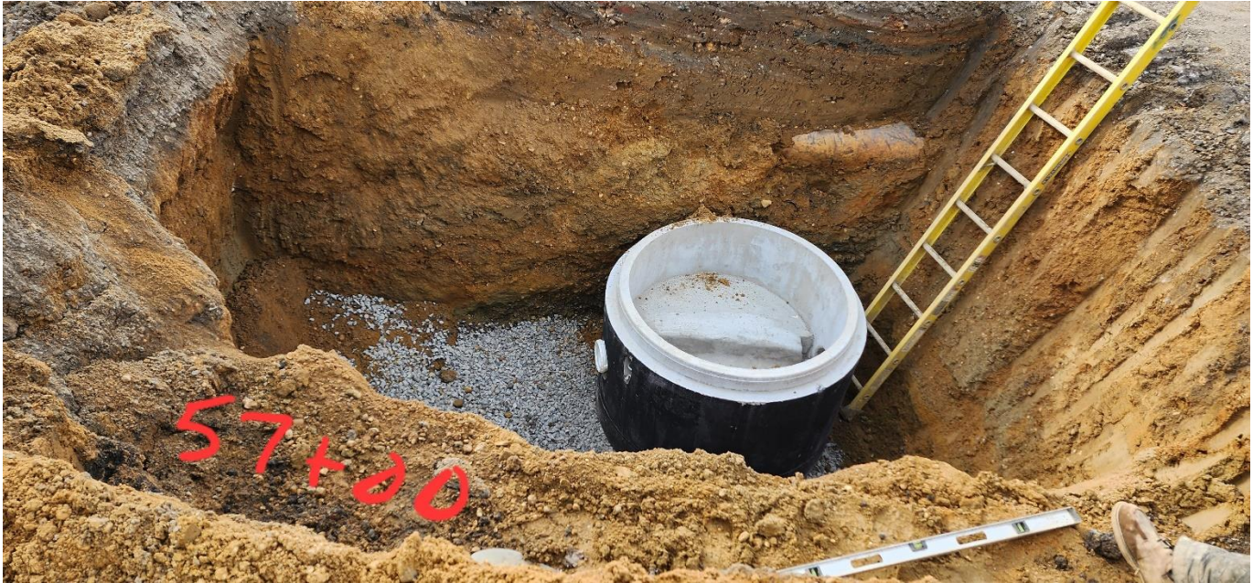
Figure 4: New sanitary manhole installation
