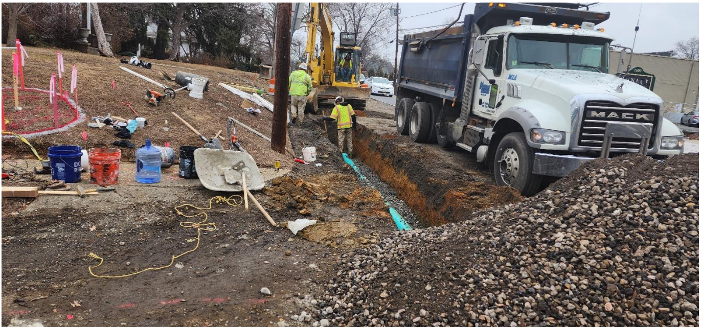
Figure:1 Sewer main installation in progress
