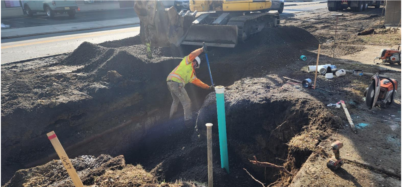
Figure 2: Sewer lateral replacements
