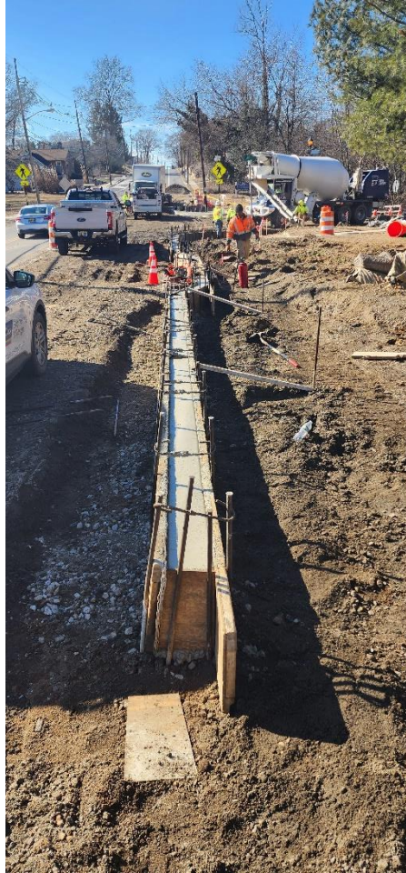
Figure 3: Concrete curbing installation in progress
