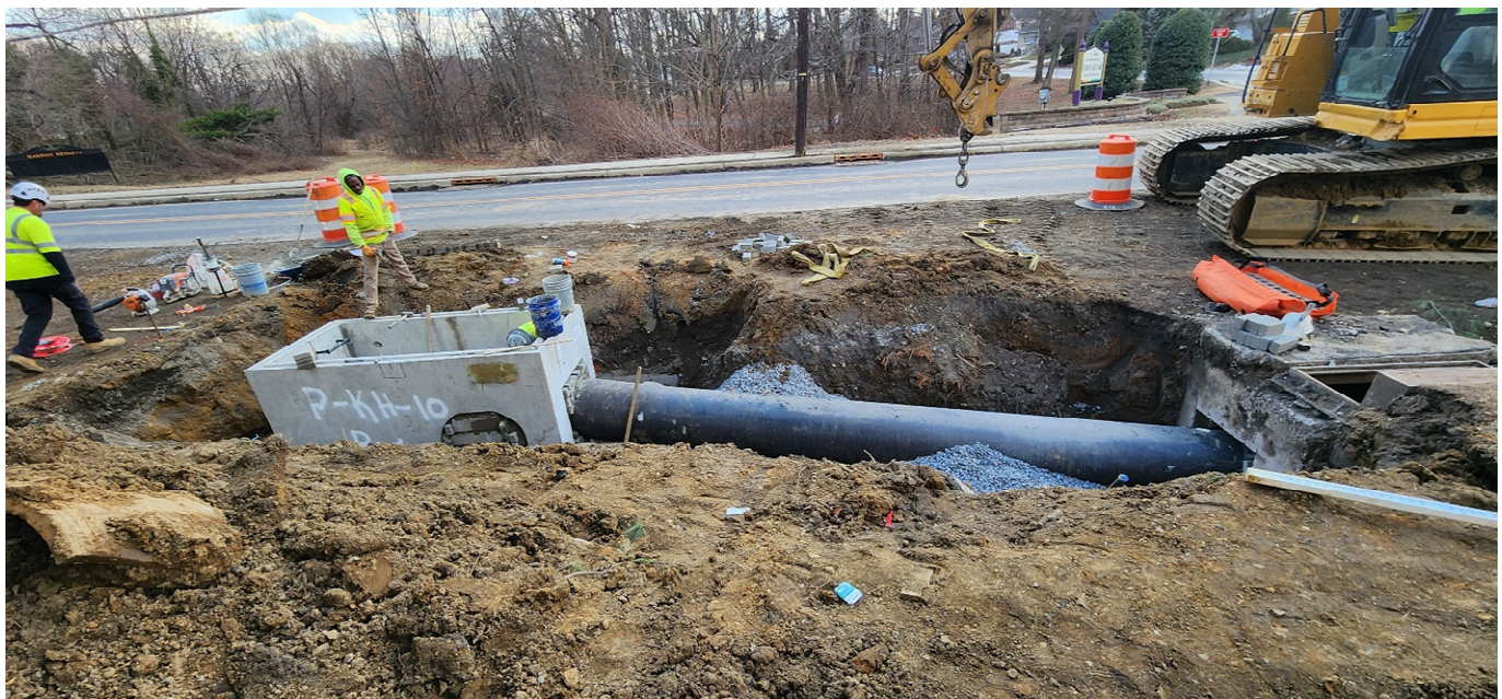
Figure 3: Inlet and drainage pipe installation in progress
