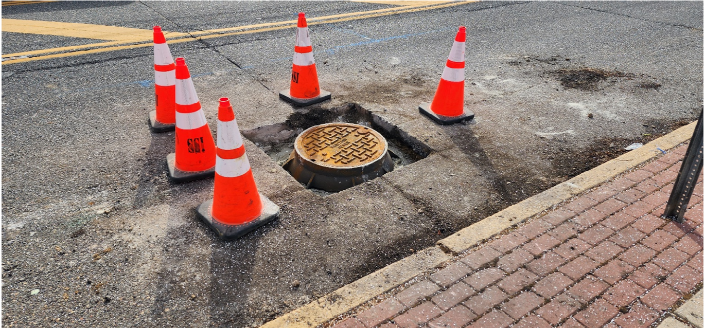
Figure 4: Manhole casting and cover replacement along segment 1.
