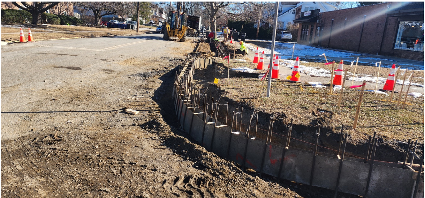
Figure:1 Concrete curb installation
