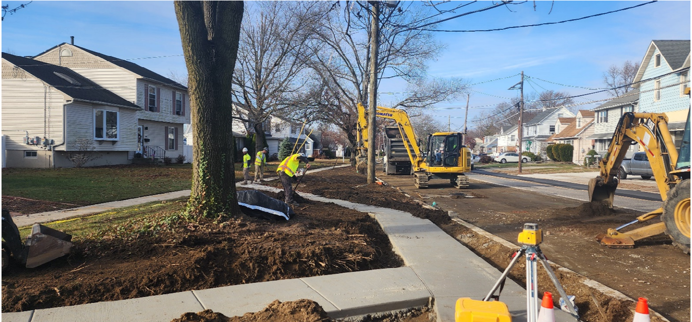
Figure 2: General site restoration
