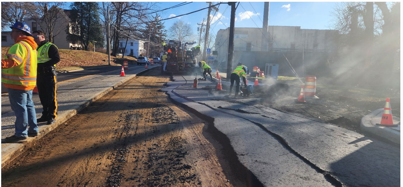
Figure 3: Paving operations along the eastbound lane of segment 3
