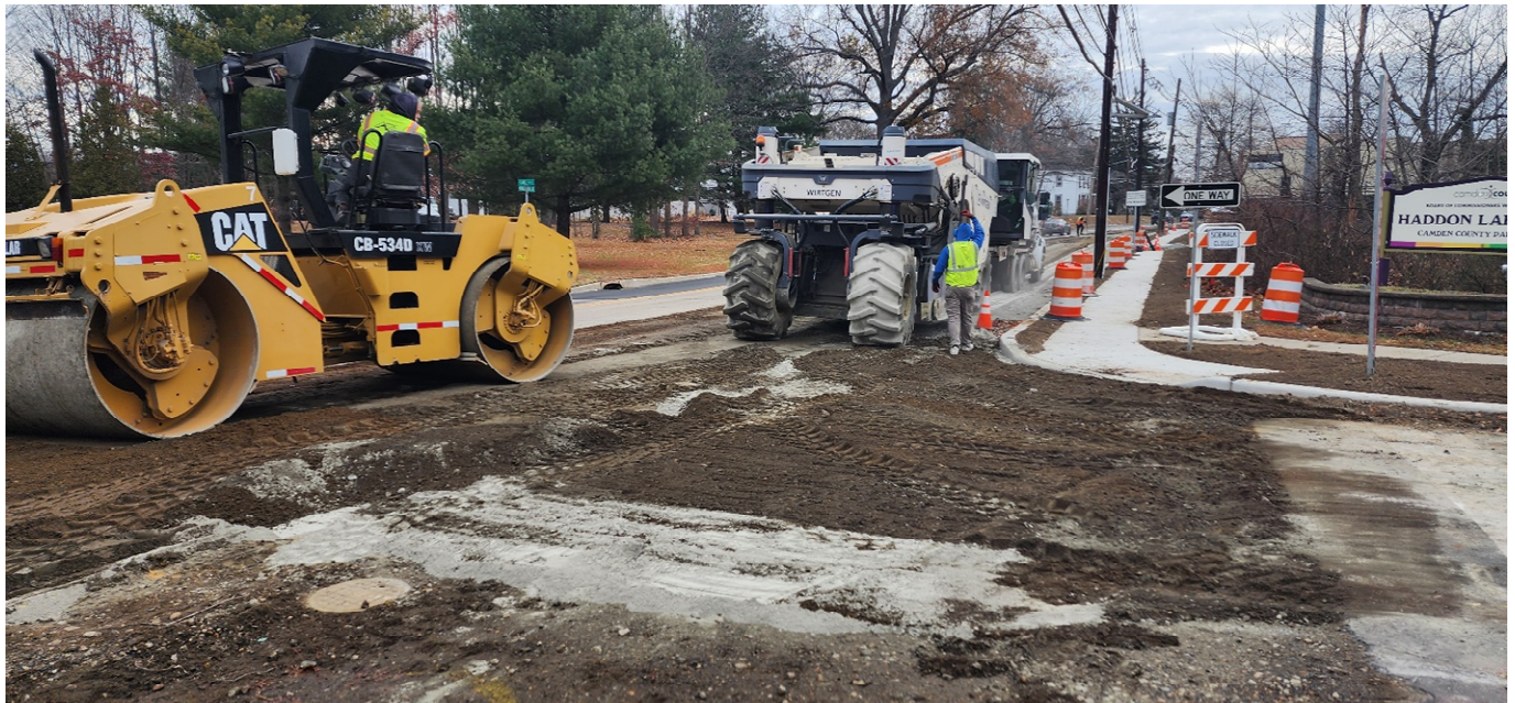
Figure 3: Began Full depth reclamation operations along the eastbound lane (segment 3).
