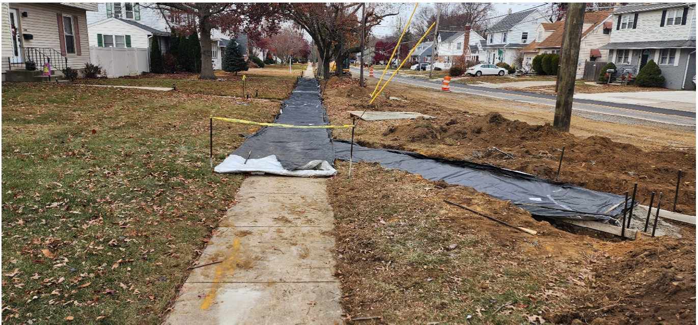
Figure:1 Continued with sidewalk, curb, and driveway installations.
